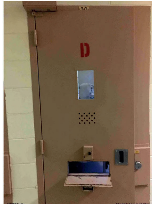
Dixon Correctional Center - Cell in mainline restrictive housing unit
