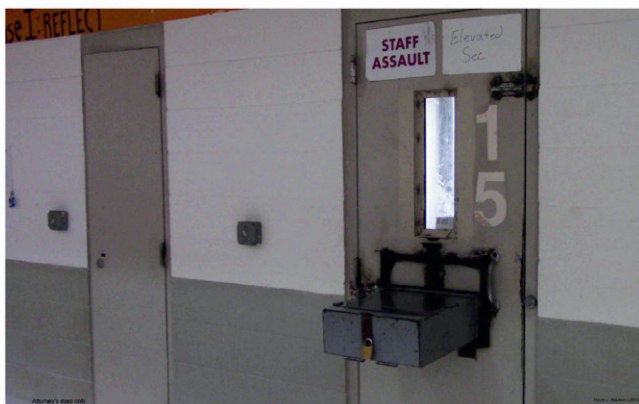
Logan Correctional Center - Restrictive housing cells in Building 15
