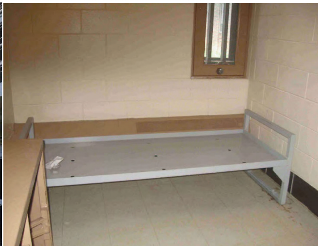
Dixon Correctional Center - Cell in mainline restrictive housing unit
